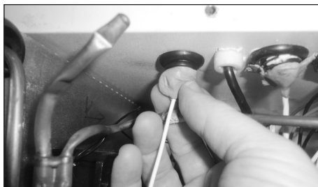
9. Closed the port hole by using putty
