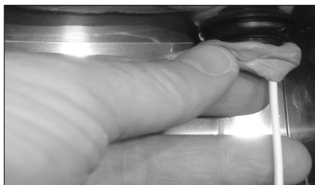
10. Close the inside hole by using putty
